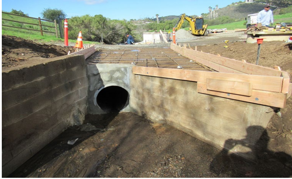
Figure 14 – January 2023 Storm – Rebuild Culvert Crossing
