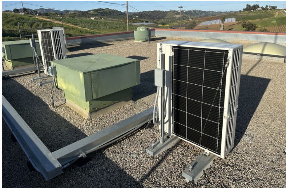
Figure 15 – Valley Center Pump Station VFD AC
