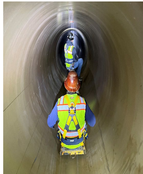
Figure 7 – Internal Pipe Inspection
